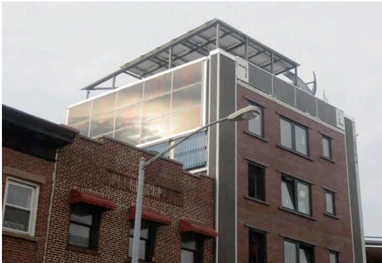
Figure 16: The Delta building in Brooklyn, NY rooftop elevated solar racking
