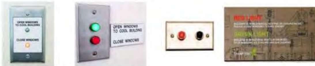
Labeled “open”/”close” indicator lights
