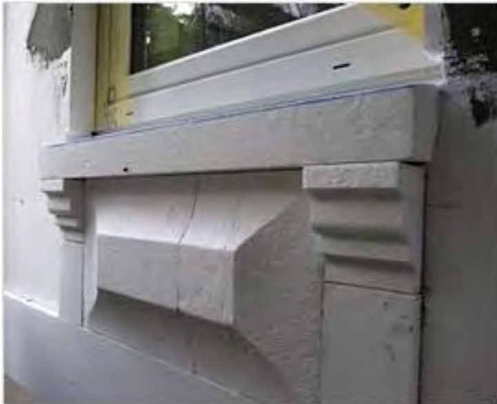
Figure 41: Brooklyn Passive House Installing EIFS
