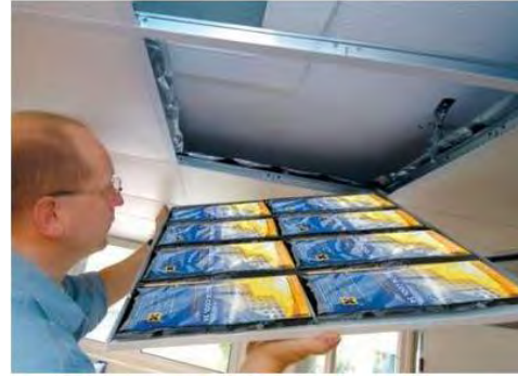
Figure 13: Installation of PCM in Ceiling Panels
