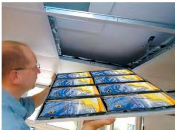
Figure 34: Installation of PCM in Ceiling Panels
