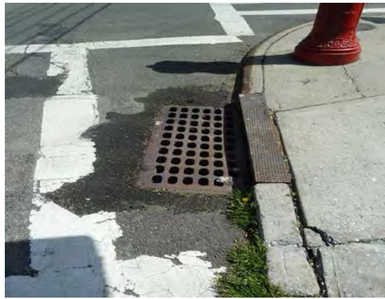
Re-pavement around the catch basin.
