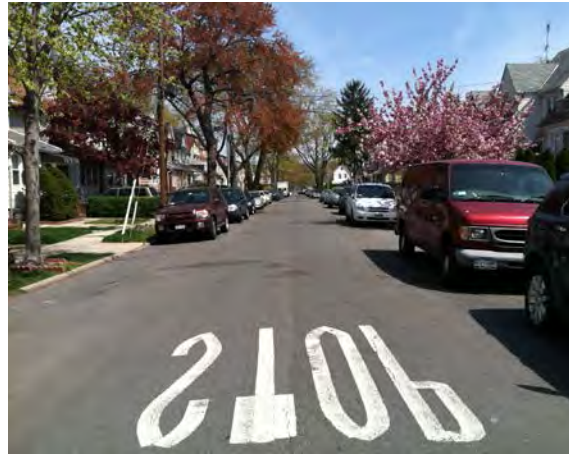
Cracks and wear-outs on the road
