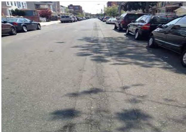
Cracking roadway
