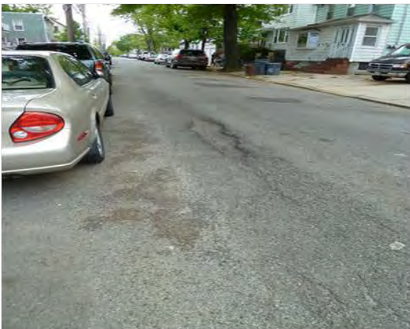
Roadway cracking
