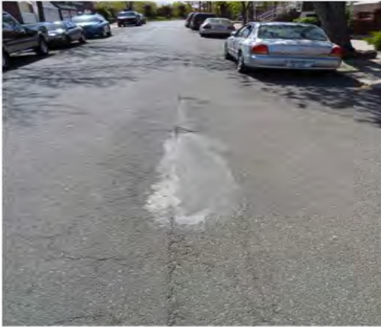
Repaving of cracked asphalt
