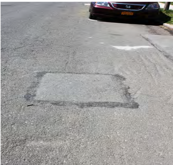
Grooving and natching in street
