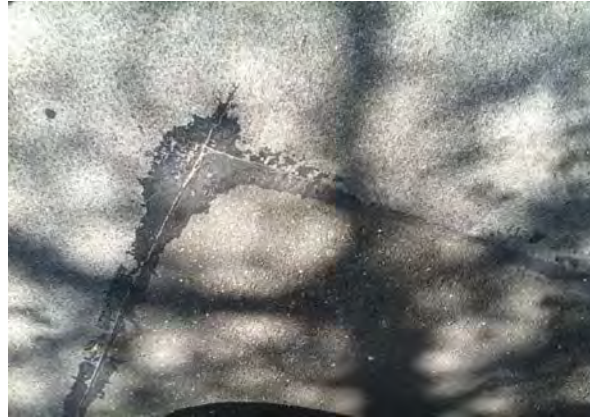
Asphalt re-pavement on the road.
