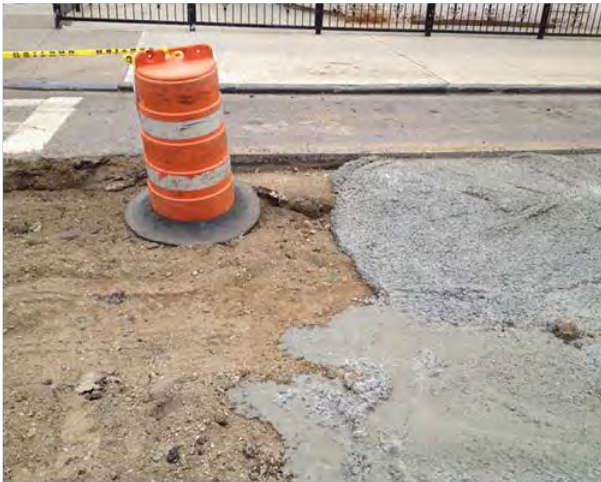
Utility backfill
