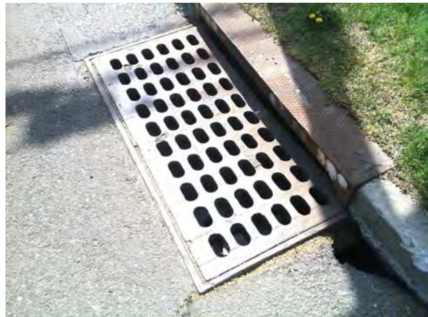
Catch basin in a generally good
