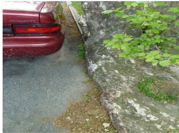
Tree impeding on roadway
