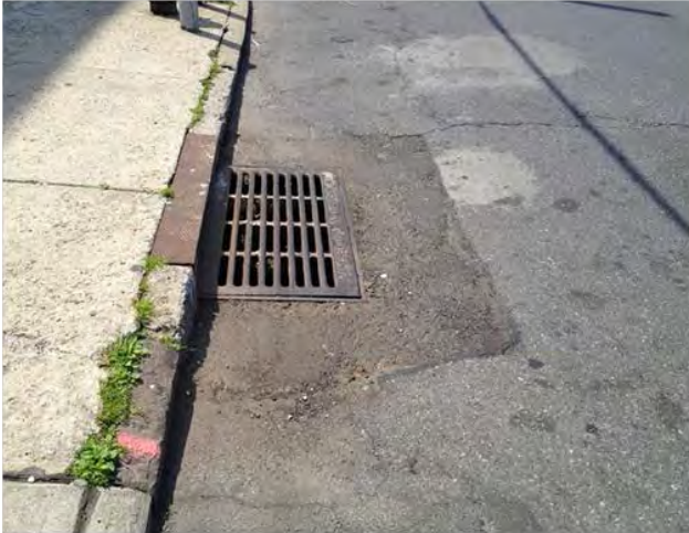
Re-work around catch basin
