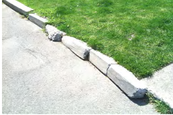
Segmented curbs around the lawn.
