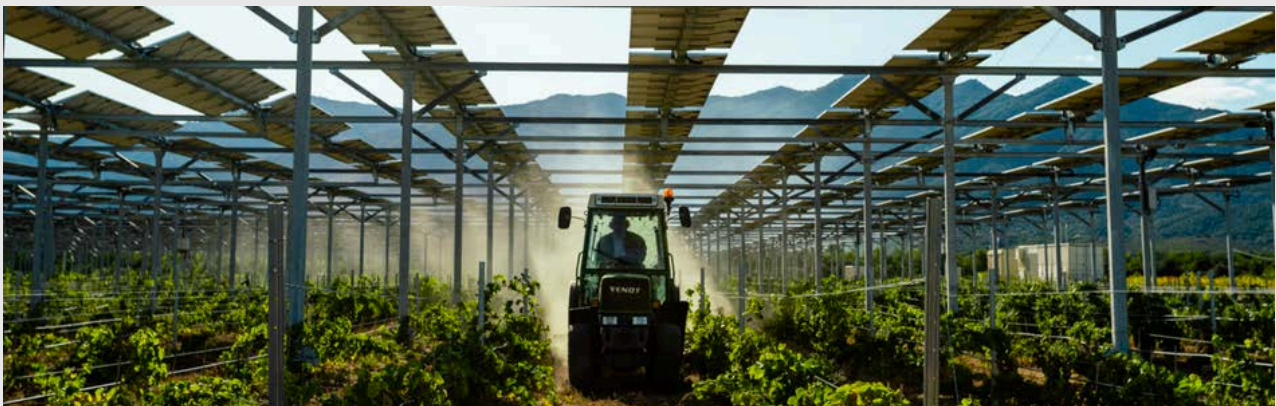
Figure 3. A tractor passing through agrivoltaics at Domaine de Nidolères, Treserre, France Source: Martin-Cocher, 2022
